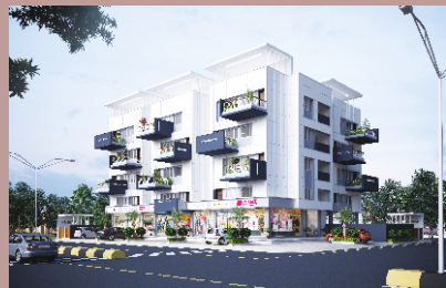
Creative Homes AURAA Katol Main Road, Nagpur
